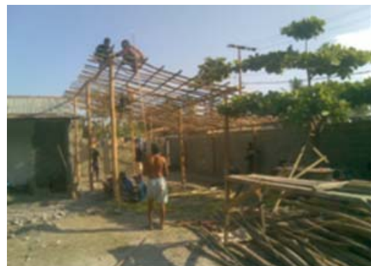
Renovation works for the classroom
