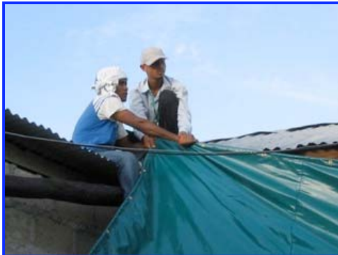
Placing canvas roof for the new classroom
